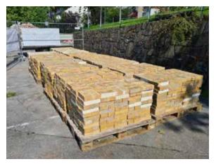
Bricks from the old building are being reused as interior cladding on several walls in the new structure.
