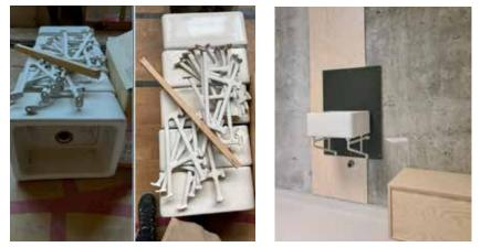
The old sinks have been preserved throughout the project and installed in new locations to function as drinking stations. Greenhouse: The previous roof structure has been dismantled and used as a greenhouse in the outdoor area. The wall on the short side facing north is covered with recycled metal sheets. The door leading to utility areas could not be used in its original location, so it was reused in the greenhouse.
