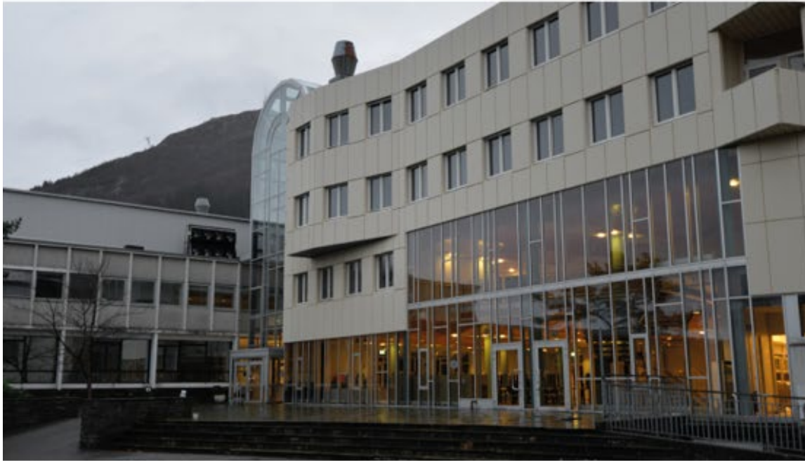
Existing facade building A
