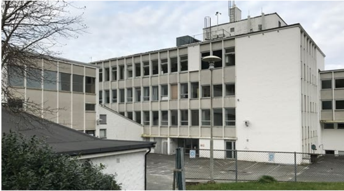
Existing facade building D
